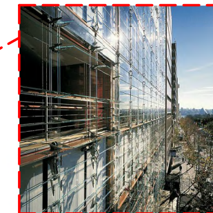
(LV(G)) GLASS LOUVRES LIGHT GREY TINTED GLASS LOUVRES (TO MATCH GL02)
